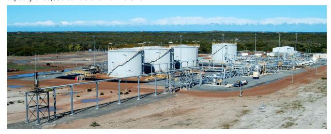
Figure 1: Arrowsmith Stabilisation Plant. Note the two outer tanks will be refurbished
